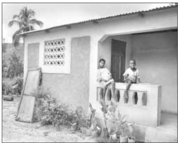
■ Ennaude says the new concrete house with a corrugated metal roof has meant a drier and better life for her family.
